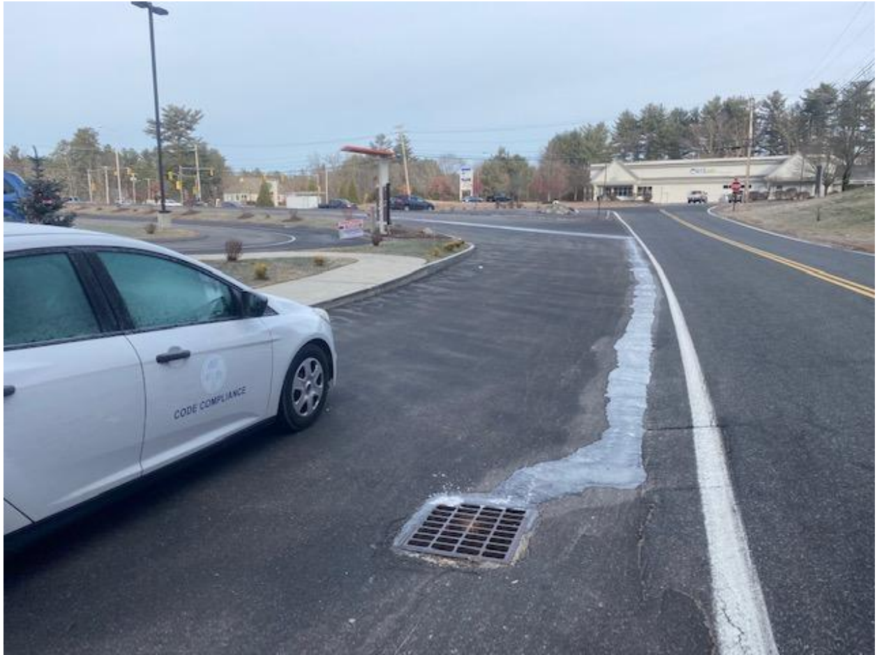
Figure 2. Flow from Manhole A. into catch basin.
