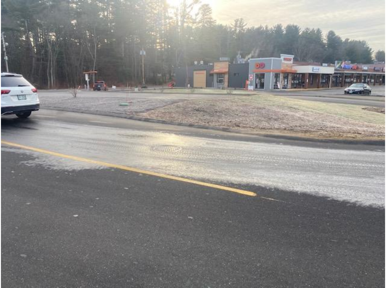
Figure 6. Centered on Manhole B. with iced flow on both sides horizontally.
