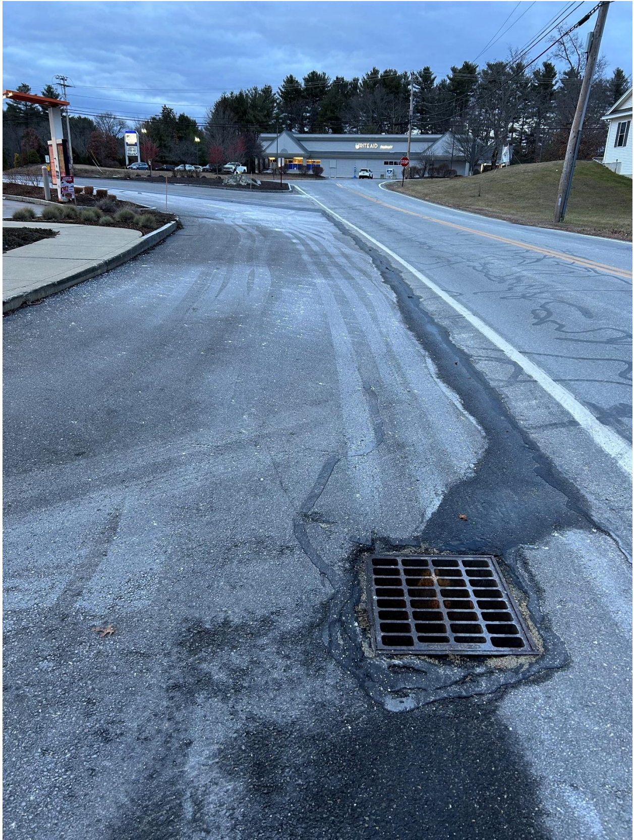
Figure 21. Flow path into the catch basin on Livingston Road.
