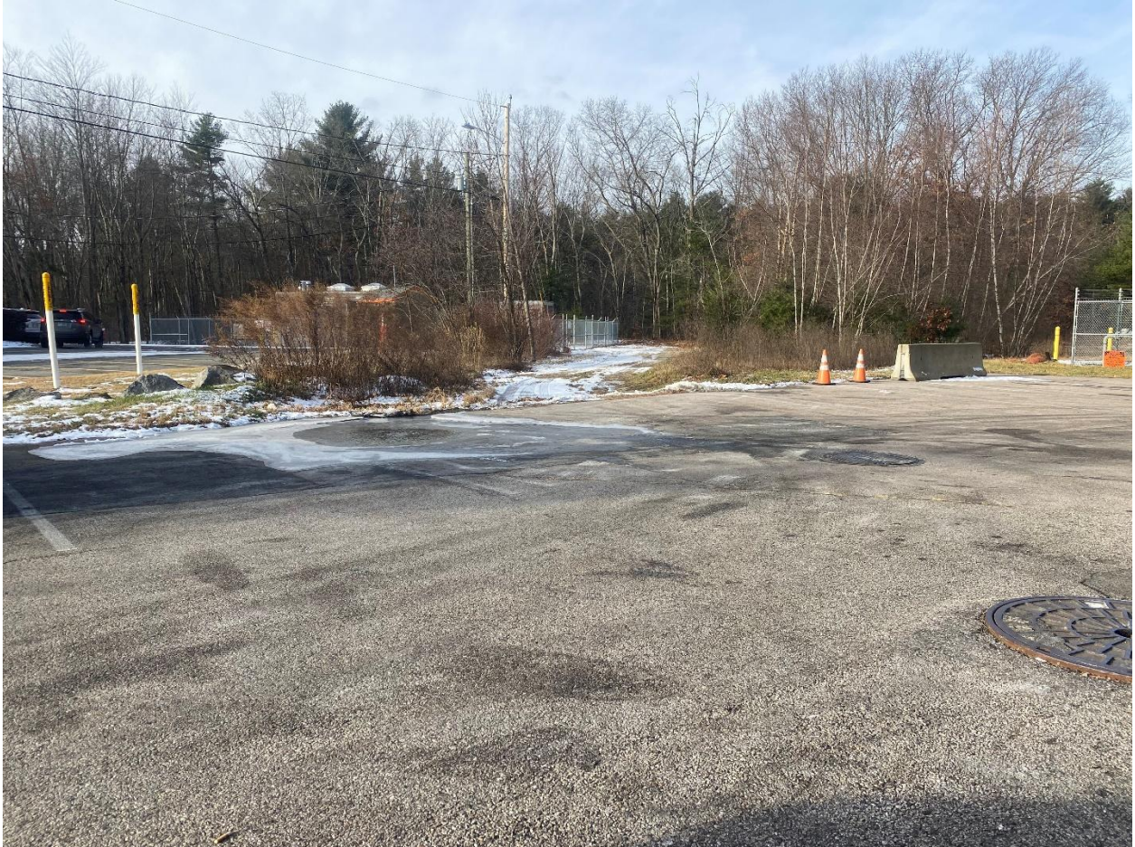
Figure 32. The septic puddle and leaking manhole.
