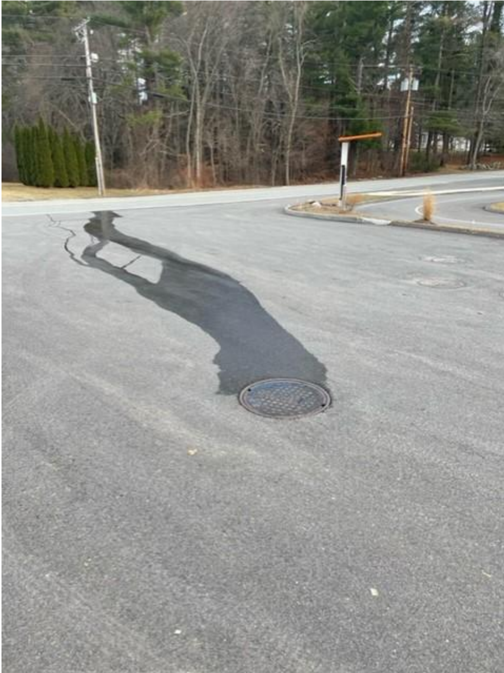
Figure 1. Sewage overflow from manhole. Picture provided by the resident.
