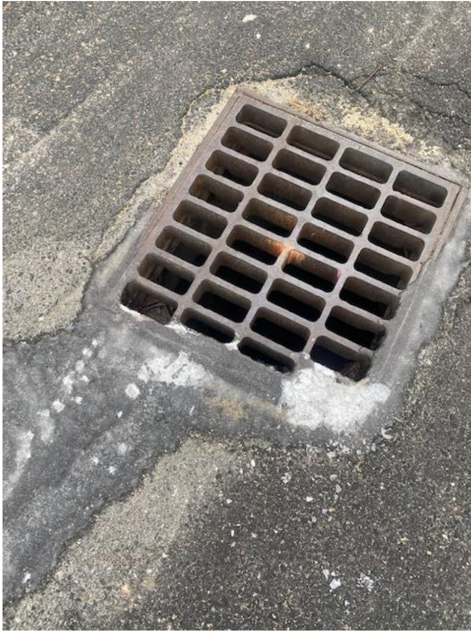
Figure 3. Close-up of catch basin that received flow from Manhole A. This catch basin empties into Tony's Brook.
