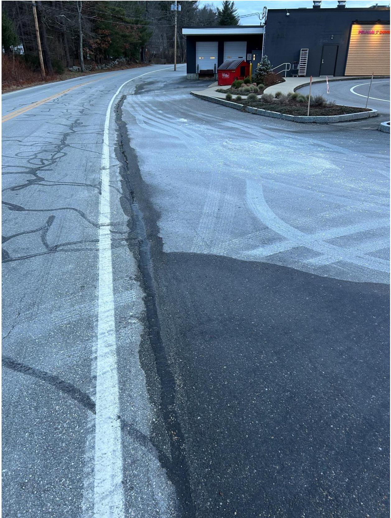
Figure 22. Flow path behind Dunkin' to the catch basin on Livingston Road.
