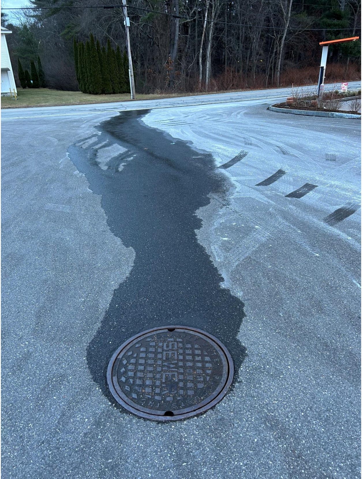
Figure 23. Overflowing manhole, facing Livingston Road.
