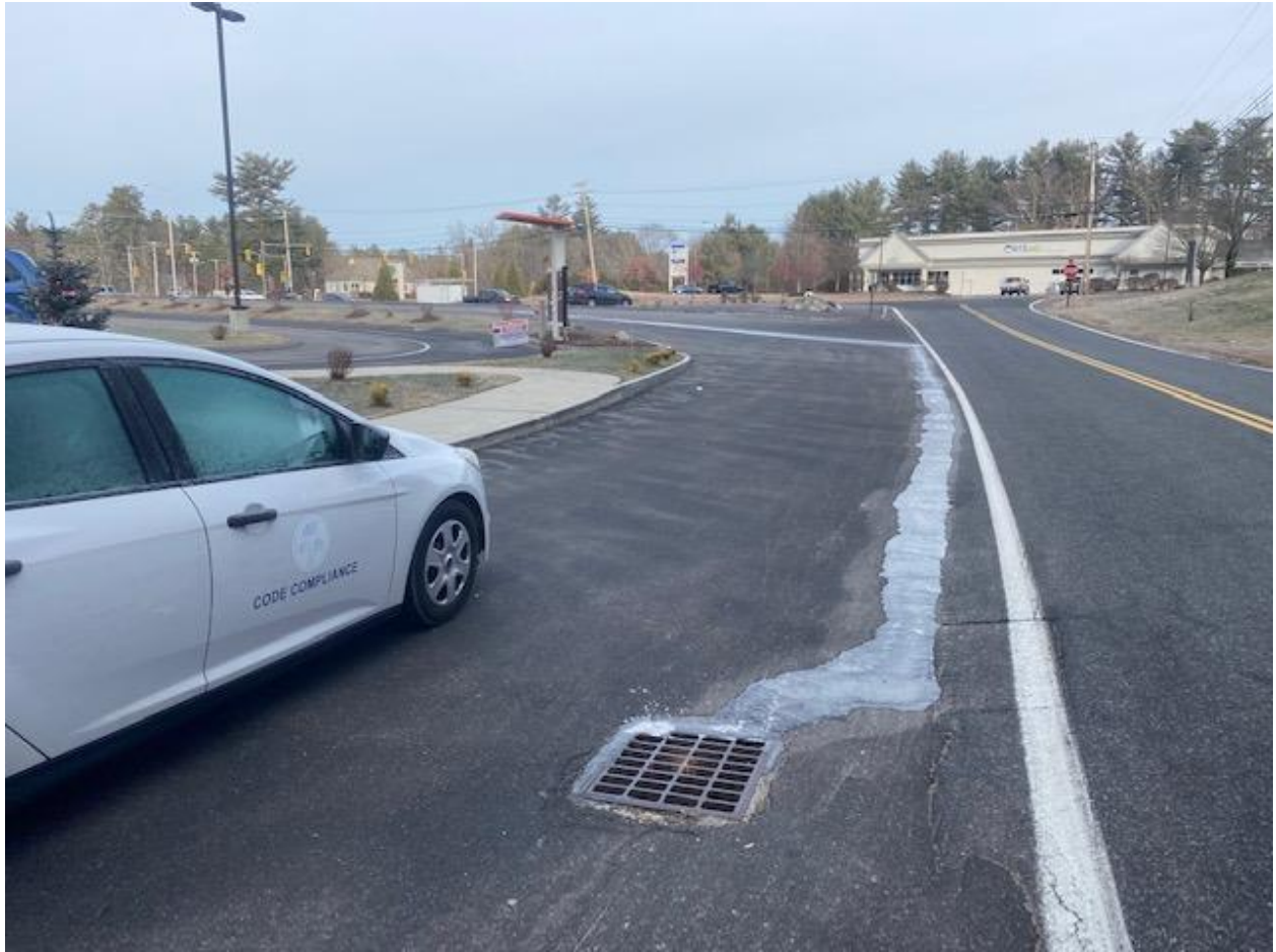
Figure 2. Flow from Manhole A. into catch basin.
