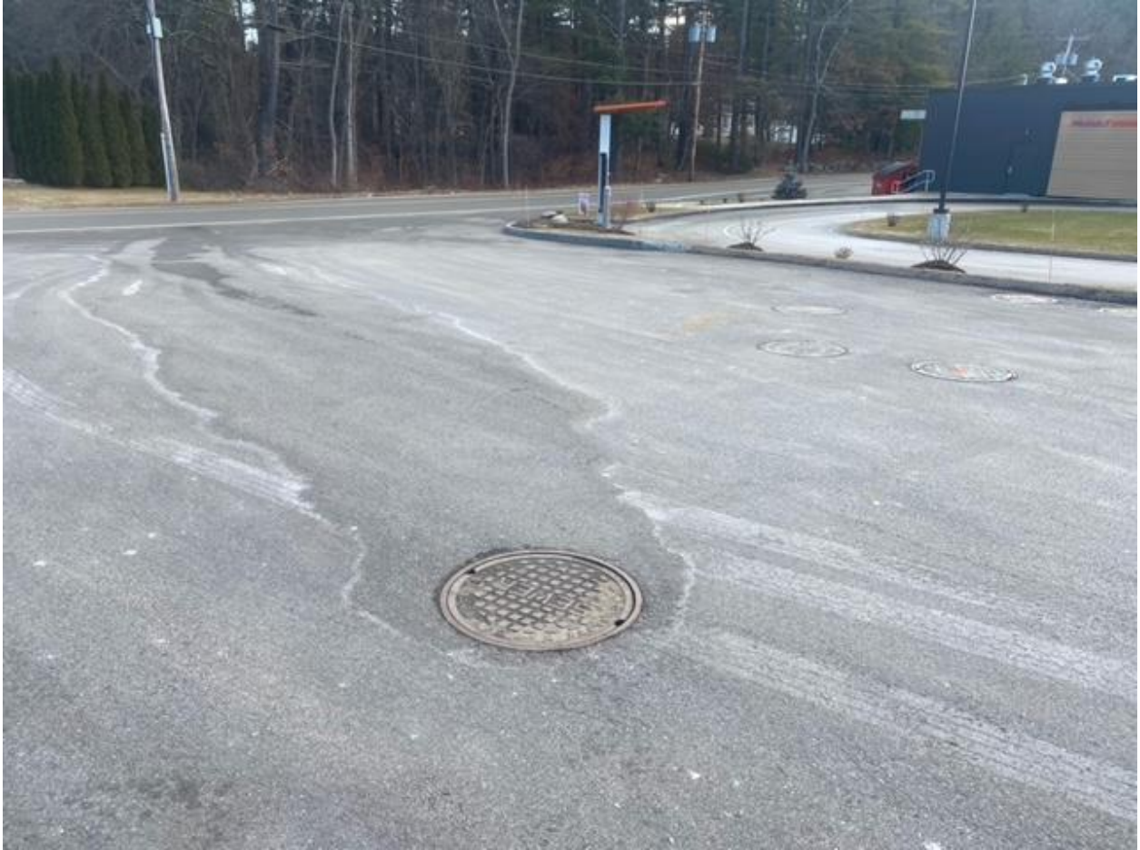
Figure 2. Manhole cover with salt-outline indicating potential overflow toward Livingston Road.
