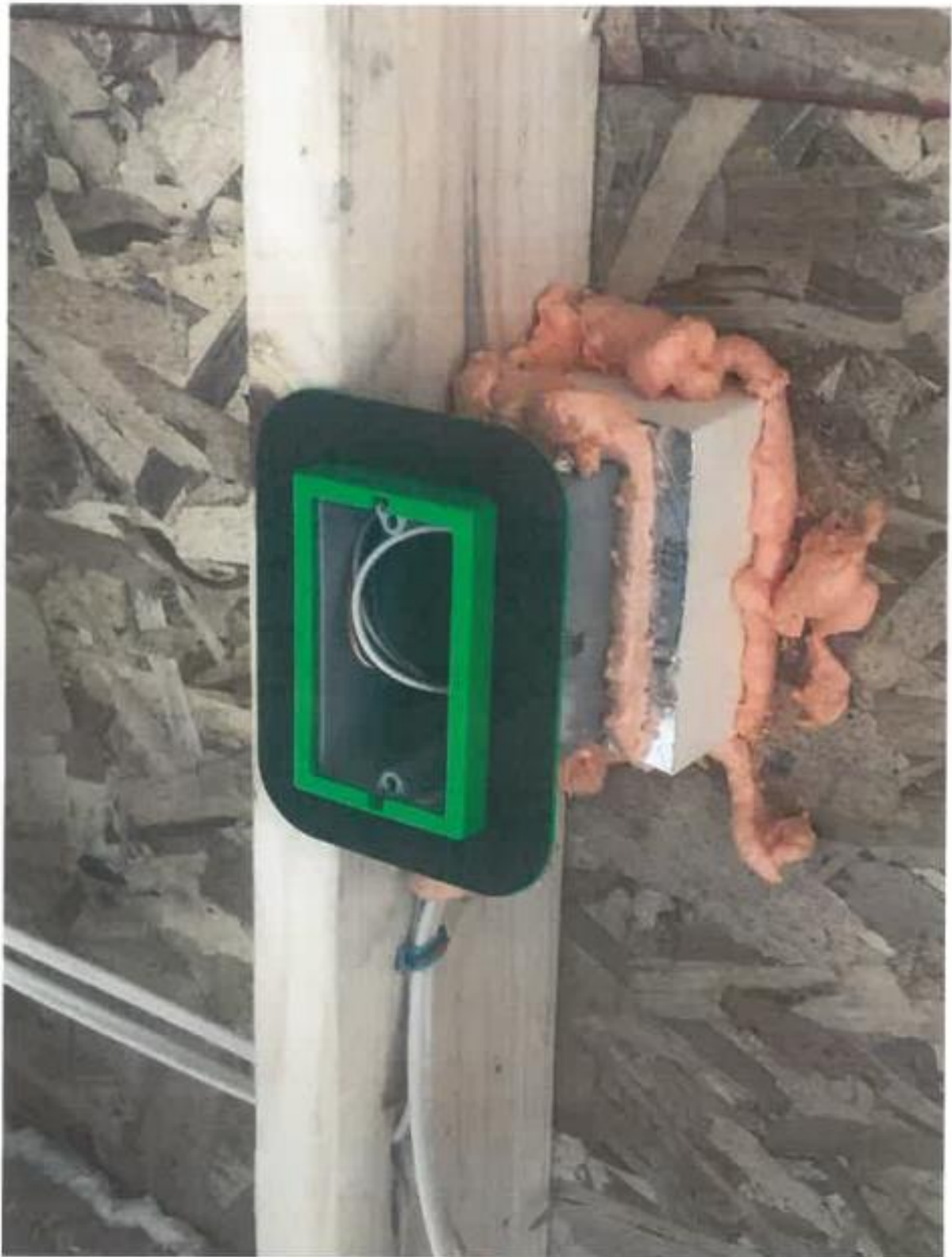
How to prevent cold air from entering a device box on exterior wall.
