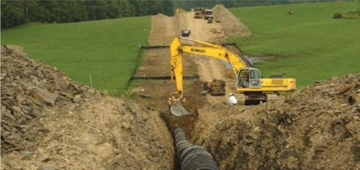
FIGURE 7: LAYING PIPE.
