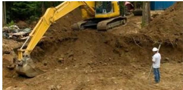
A qualified representative from Kinder Morgan must be on site whenever an excavation is underway or equipment is being used within 25 feet of our pipeline or as determined by Kinder Morgan personnel and procedures.
